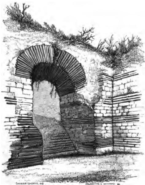
2. Porchester Castle, Hampshire. Roman Masonry and Arch formed of Roman bricks or tiles.
